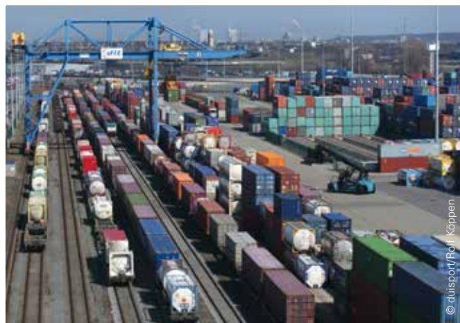
More than 3.7 million standard containers (TEU) are handled annually on a site totaling 1550 hectares.
