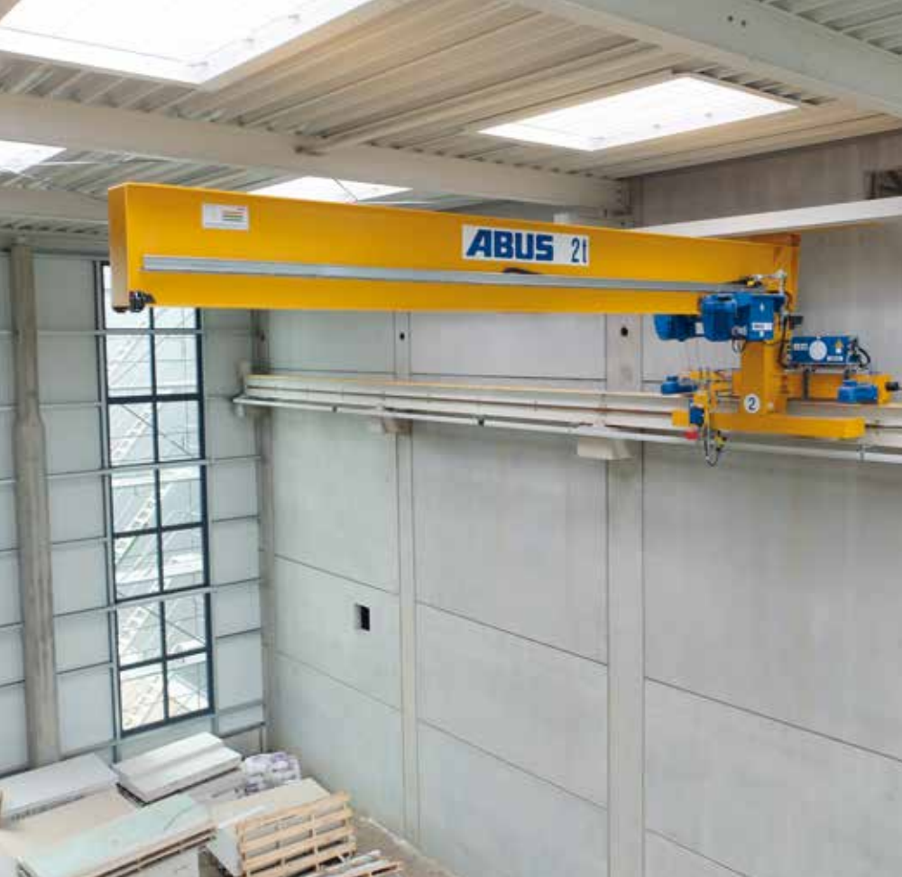
The new technology centre: The crane is already suspended
