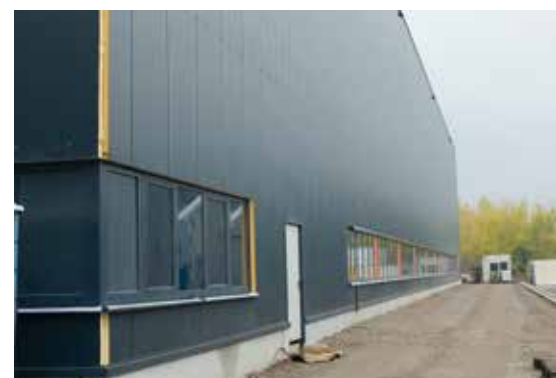
Sideward view of the new construction
