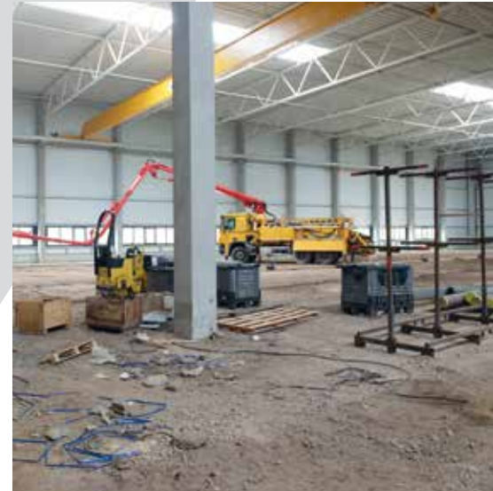
The interior view of the new production hall
